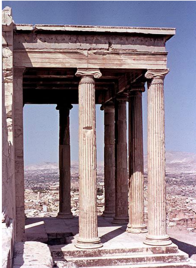
In the northern hall of the Erechthion Poseidon's trident was kept.
